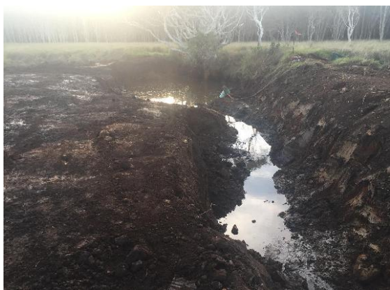
Plate2: All asbestos impacted bulk refuse and soil removed back to natural. No visible ACM remains.
