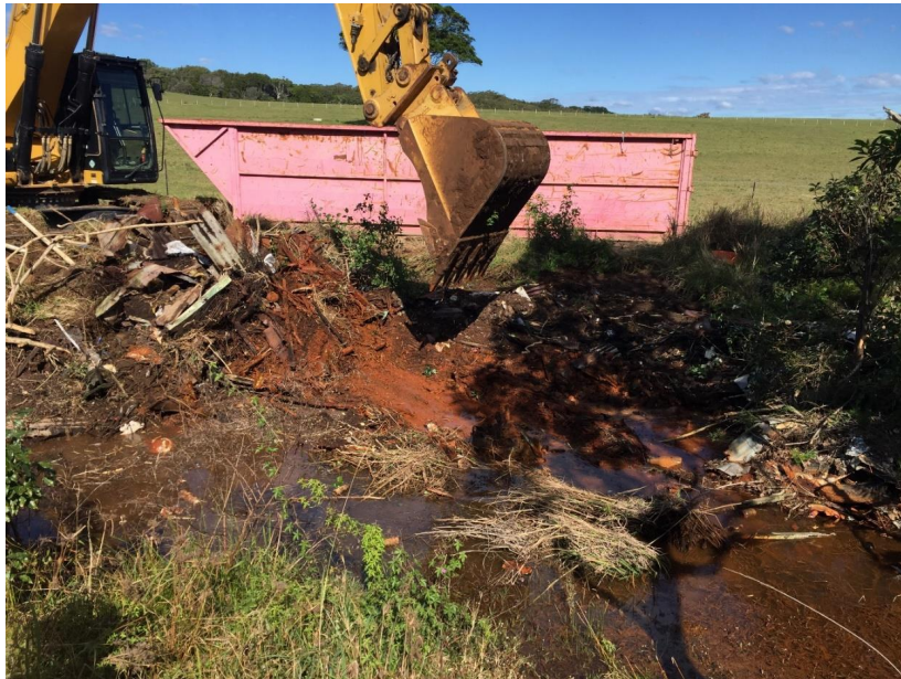
Photograph 5: Water ingressed into the pit, mostly from the upslope end, occurred in the pit as excavated progressed
