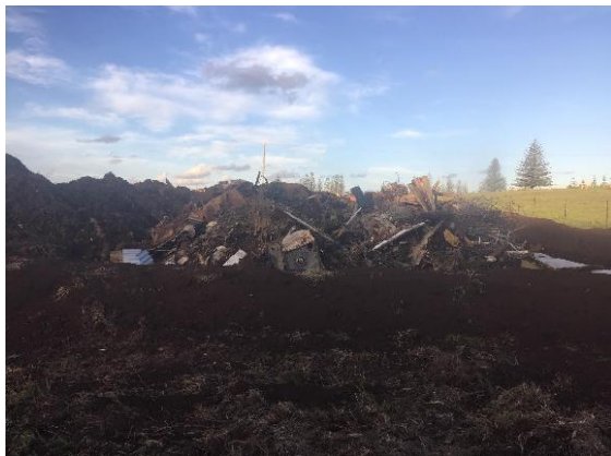
Plate1: Asbestos impacted material (bulk refuse) removed and stockpiled on geofabric until disposal permit granted.
