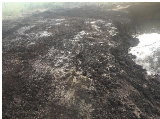
Plate2: All asbestos impacted bulk refuse and soil removed back to natural. No visible ACM remains.
