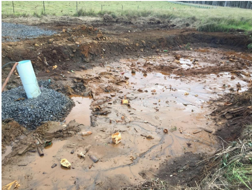
Photograph 7: View looking west-north-west across the main part of the remediation area. The pipe in the middle was used to pump out some of the water in the excavation to allow validation of the soils in the base of the pit.
