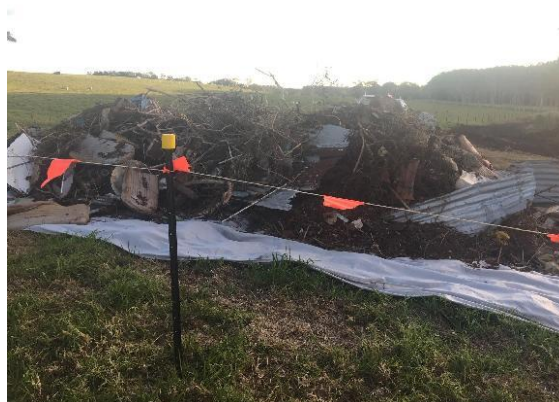
Plate1: Asbestos impacted material (bulk refuse) removed and stockpiled on geofabric until disposal permit granted.
